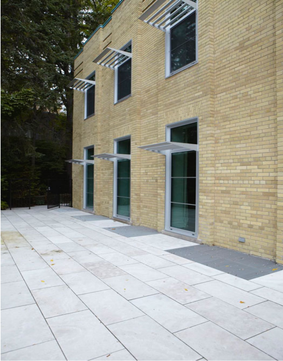
Exterior brick work with metal shades
