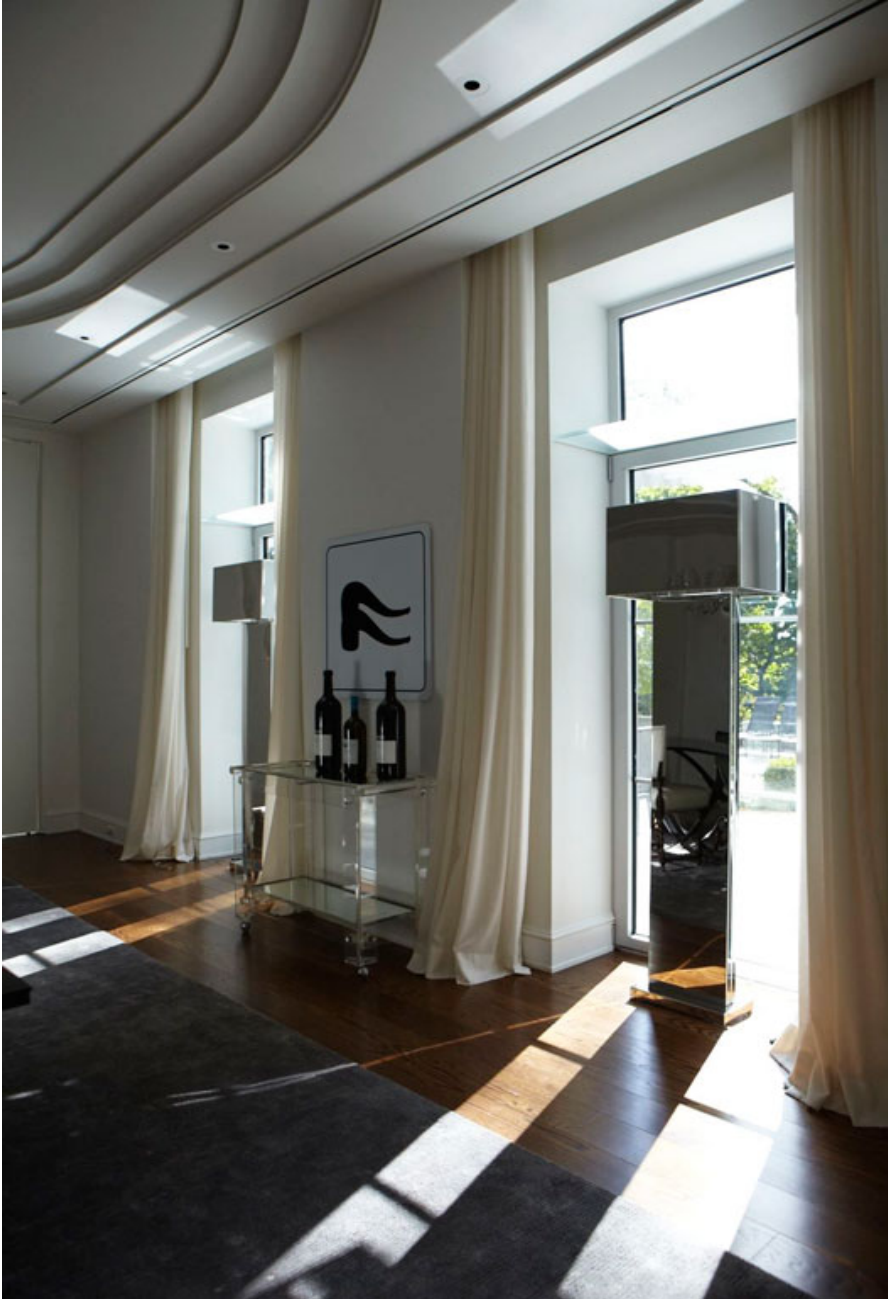
Glass light shelves visible above interior window panes
