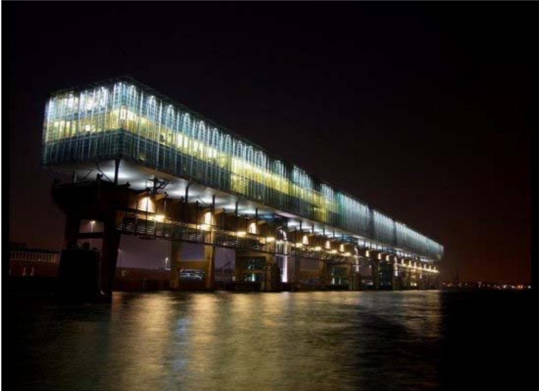
Kraanspoor means "crane track" which is what this concrete structure was when it was erected in 1952 as part of the Dutch Dock and Shipbuilding Company's facilities. Two cranes traveled up and down tracks that ran its length, while ships under construction were tied alongside it. It was abandoned in 1984 until it was repurposed as the base for a 134,549 sq. ft. glass-walled office building in 2007.
